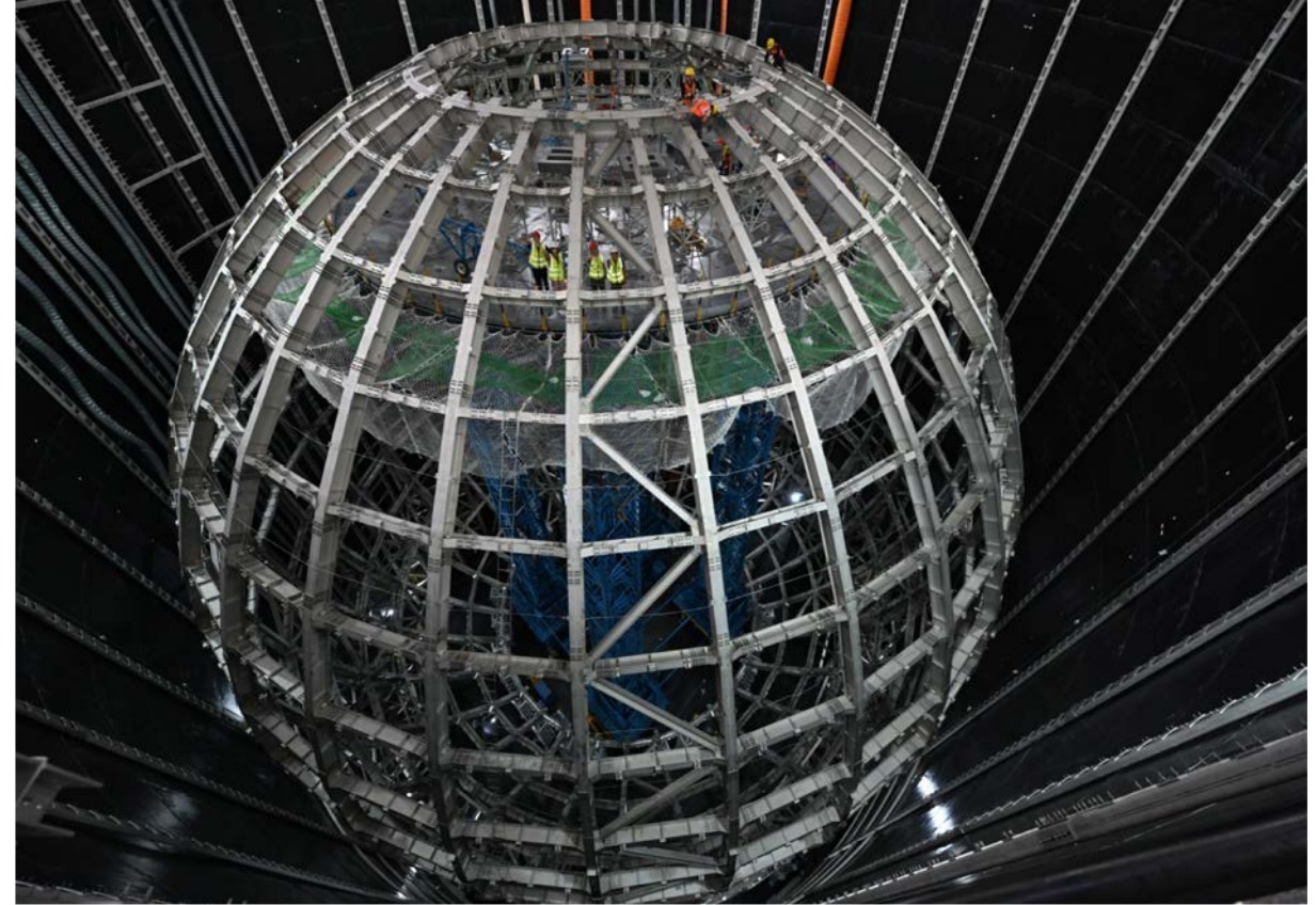
Support structure finished (June 2022)
