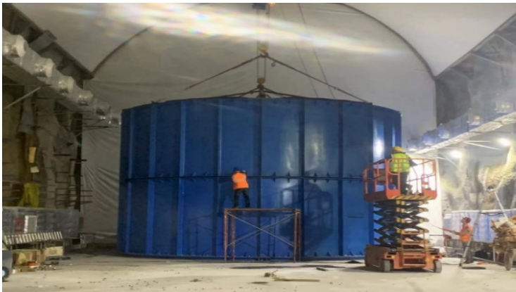
OSIRIS - LS monitor – under installation
