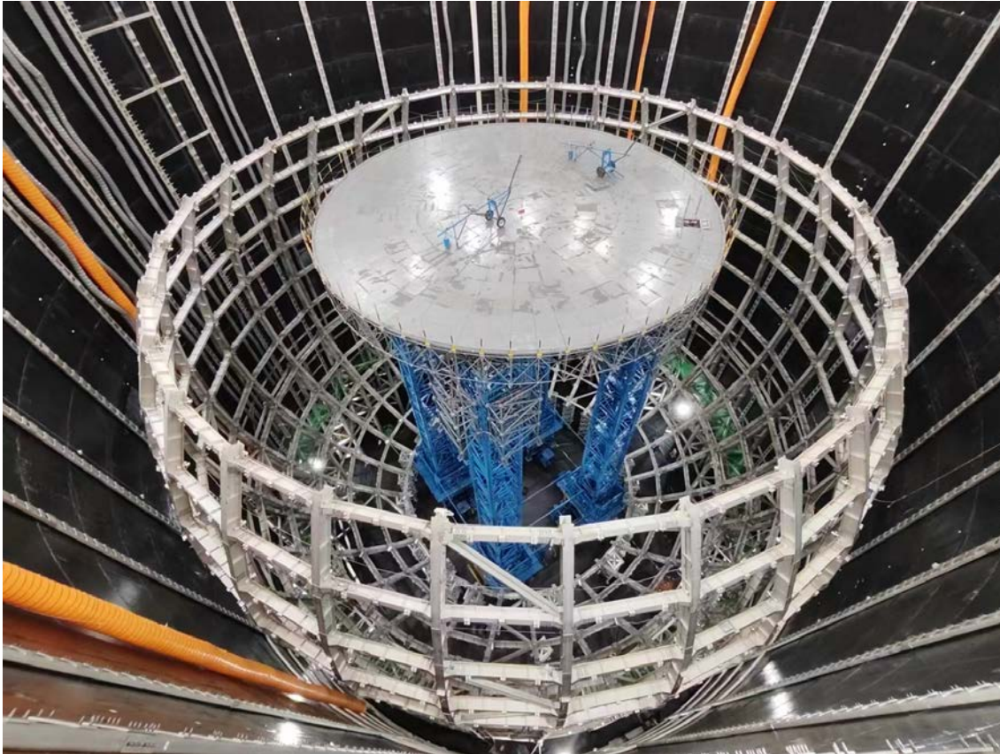
Installation platform finished (May 2022)
